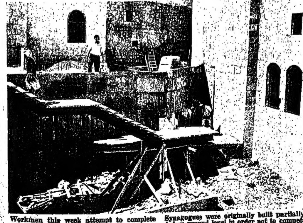
Workers this week attempt to complete main entranceway to the Sephardi Synagogue complex before next week's opening. Synagogues were originally built partially below ground level in order not to compete in height with nearby mosques.
